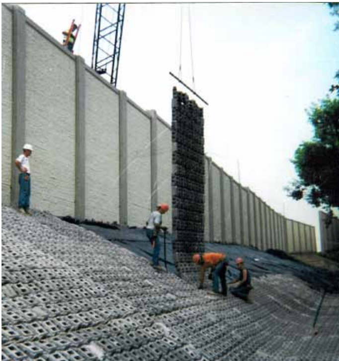
Figure 6—Cabled ACB Installation Behind a Sound Barrier
