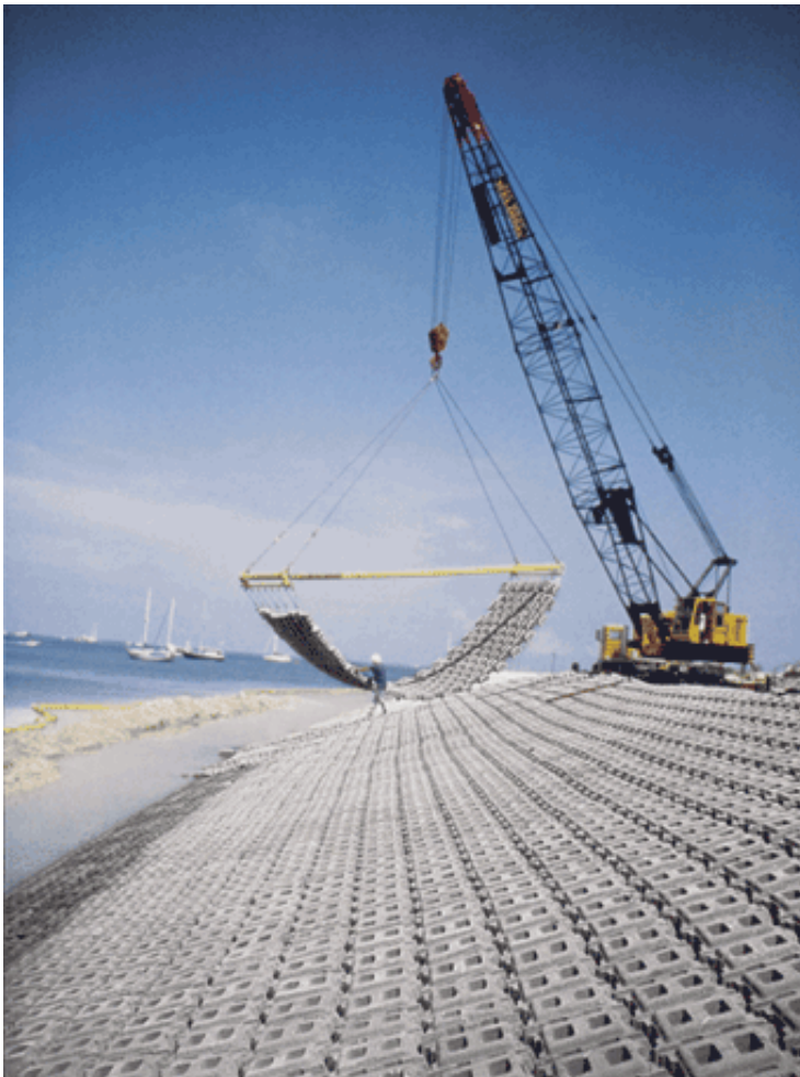
Figure 5—Placement of Cable ACB System With Crane
