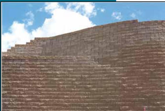
Figure 12. Partially Terraced Wall
