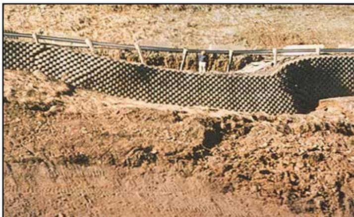
Figure 19. Global Stability Failure Example
