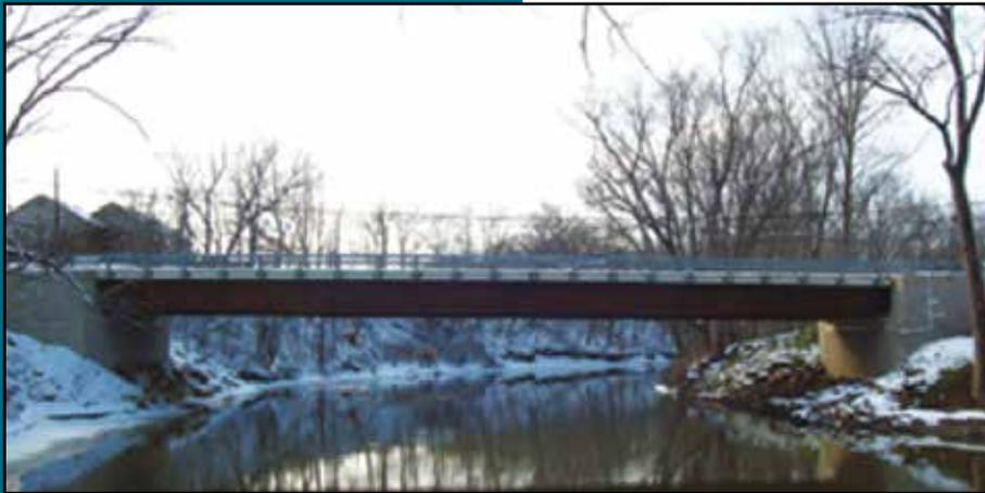
Figure 1. Geosynthetically Reinforced Soil-Integrated Bridge System (GRS-IBS) Wall
