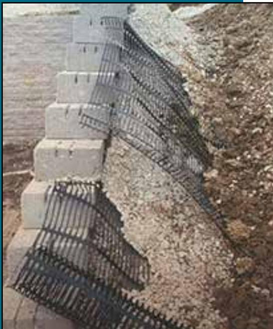
Figure 2: Poor Installation Example (The reinforcement has been installed in the wrong direction, the geogrid is not horizontal or taut, the geogrid was not installed all the way to the front of the unit, and the soil and gravel have not been compacted)
