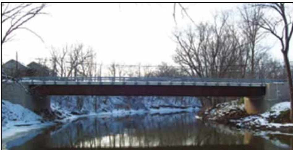
Figure 13. Geosynthetic Reinforced Soil — Integrated Bridge System (GRS-IBC) Wall
